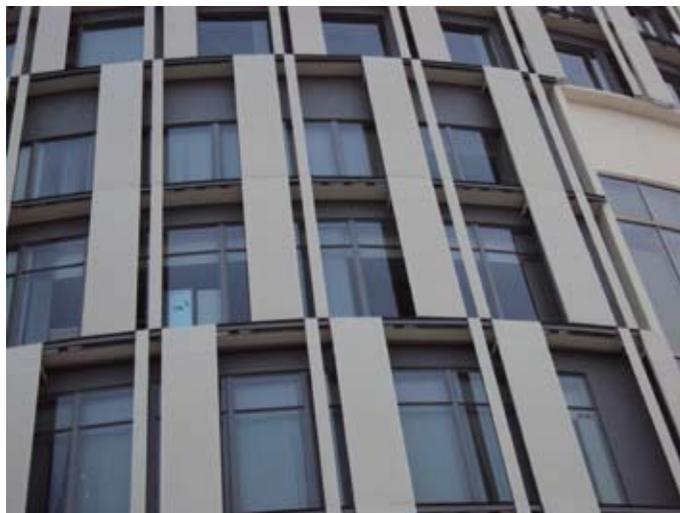
*Sun shading panel of Cheng Yu Tung Building to prevent solar heat gain*
